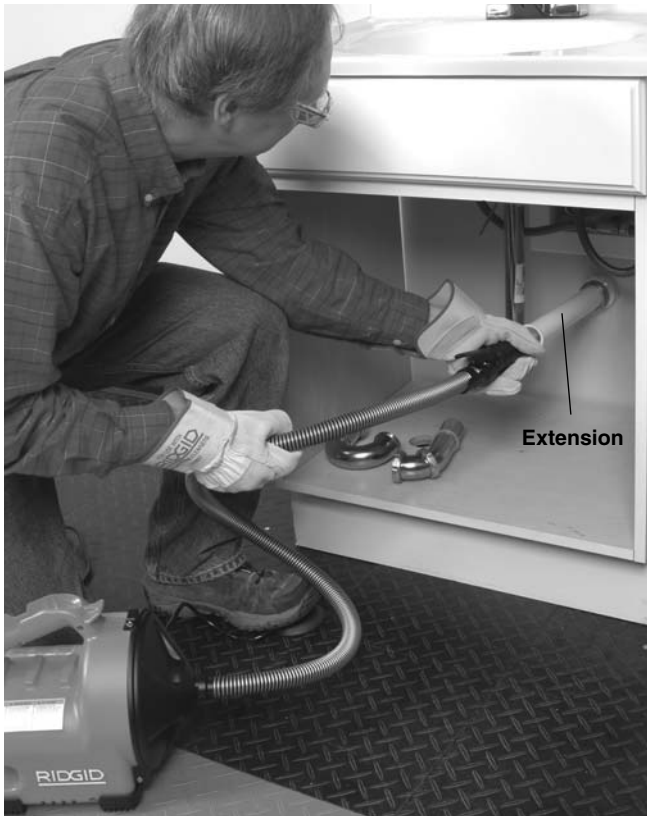
Figure 11 – Example of Extending Drain to Within 6" (15 cm) of AUTOFEED.
