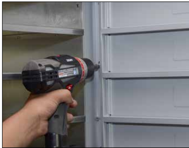
Figure 16– Secure units together using connector machine screws
