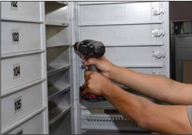
Figure 3 – Top side of unit facing wall
