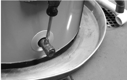
Figure 10 - Draining the old water heater.
