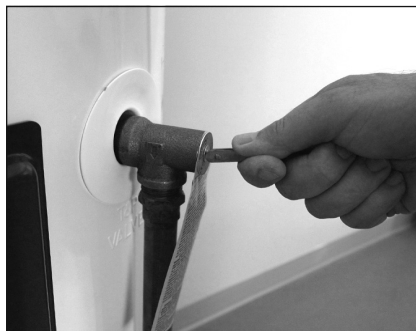
Figure 38 - T&P Relief Valve
